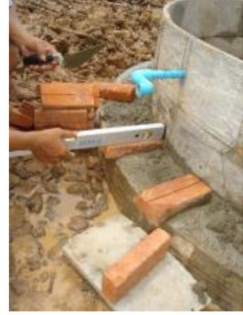
**Figure 9 – Starting the outlet tap box**
