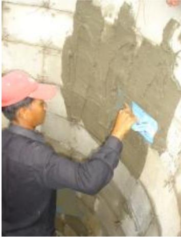
**Figure 13 - Applying the first layer of render to the inside of the tank**
