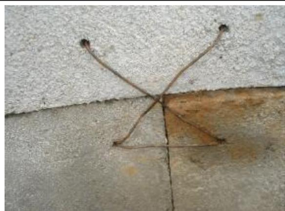
**Figure 12 - Detail of the wire ties for the cement bricks**
