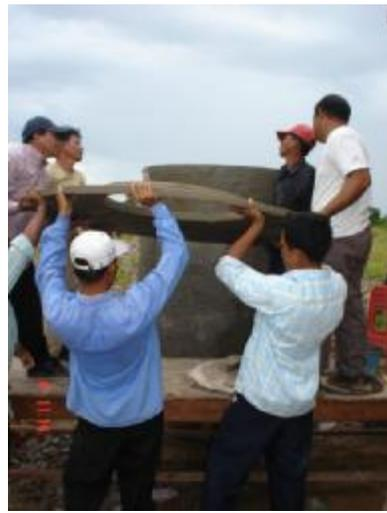
**Figure 14 - Fitting the top covers**
