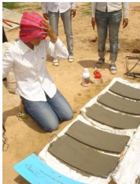
Figure 2 – Filling the cement brick moulds
