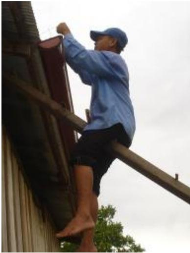
**Figure 16 - Fitting the gutter to the roof**
