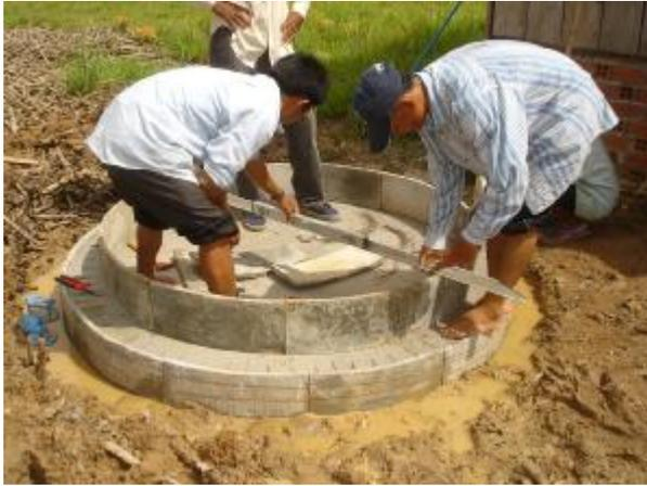
**Figure 8 – Checking level of first layer of segments**
