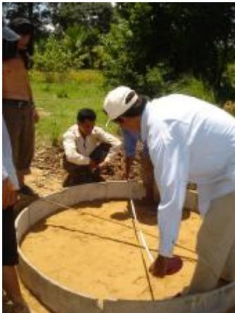
Figure 5 – Checking roundness of 12 bricks on base
